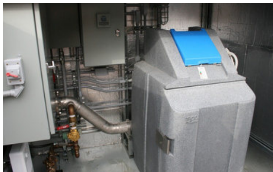
Above: Automated refrigerated sampler with auto tagging to septage hauler's account and ID
