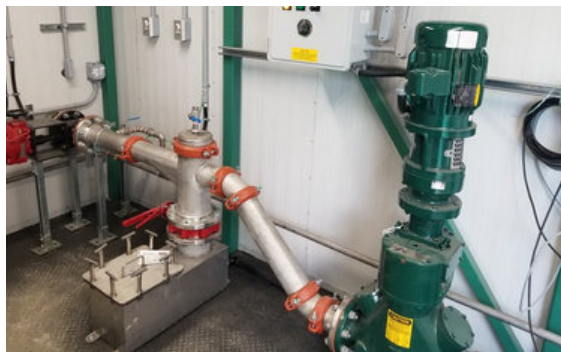
Below: Pretreatment devices integrated into stations allow for easy handling of solids such as rocks, ragging and grease
